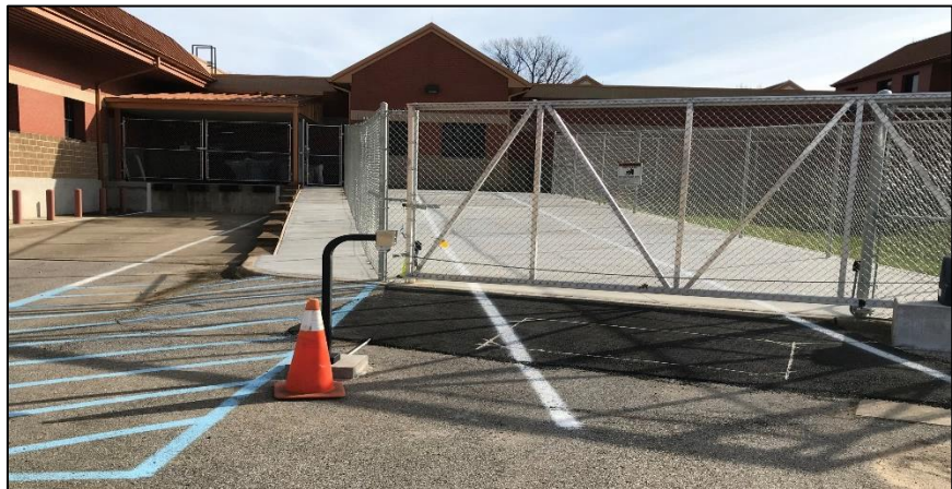
Figure 3.C JRJDC Sally Port Fencing
