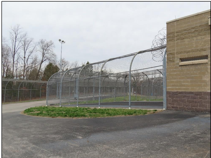
Figure 2.B Adair Regional Juvenile Detention Center Fencing February 24, 2023
